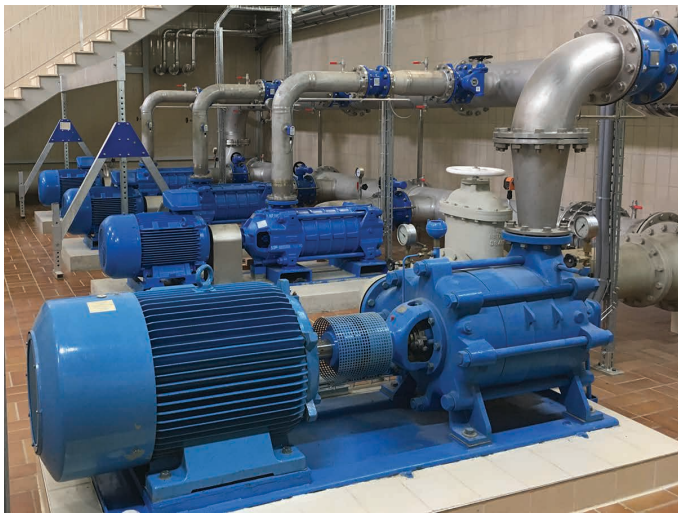
Fig. 2: The new IE4 motors are significantly more energy-efficient than standard I2 motors. The use of DG1 variable frequency drives further improves the energy balance of the system.
